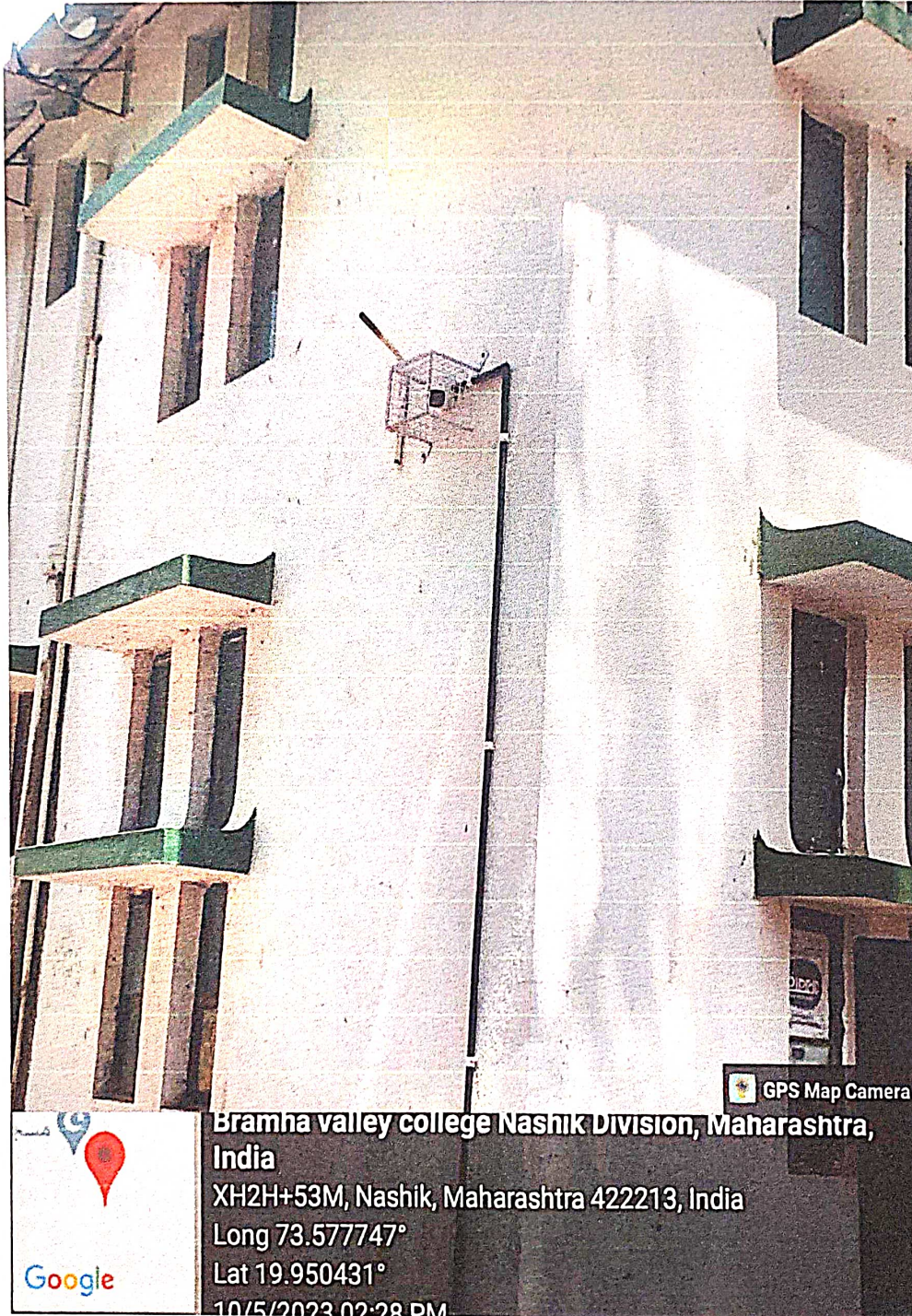
1.2 Photo: CCTV Camera at Ladies Hostel
